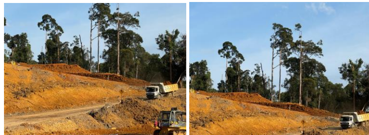
Area Operational unit : Land Clearing naik & turun Extrem area Lampunut
