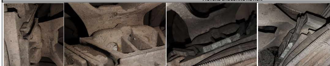
Kondisi Engine Mounting LH Front
